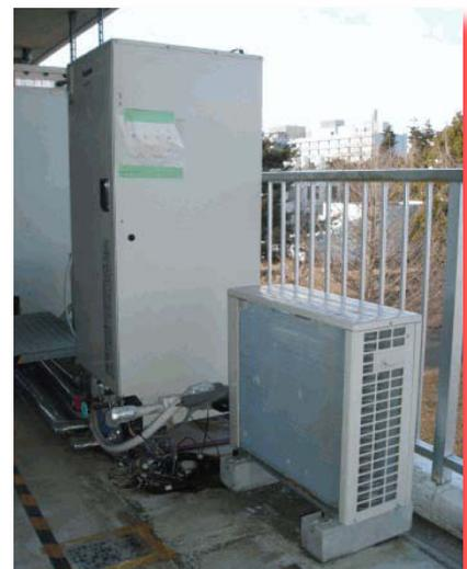
Figure 3. EcoCute - heat pump domestic hot water system.
