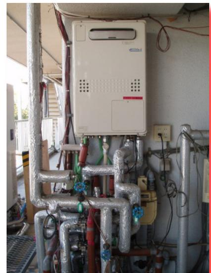
Figure 2. Condensing boiler under test.
